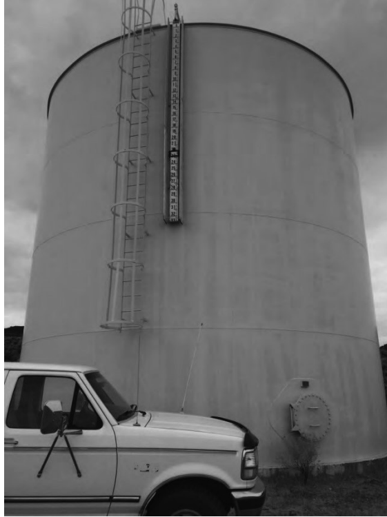
Figure 7: Image of the storage tank and water level staff gauge.
