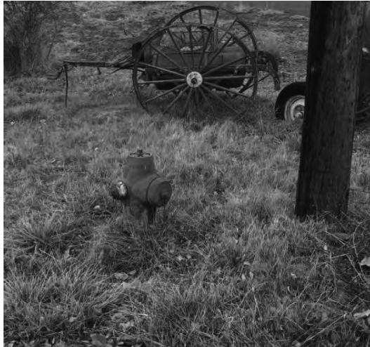
Figure 13: Image of a hydrant that does not work.
